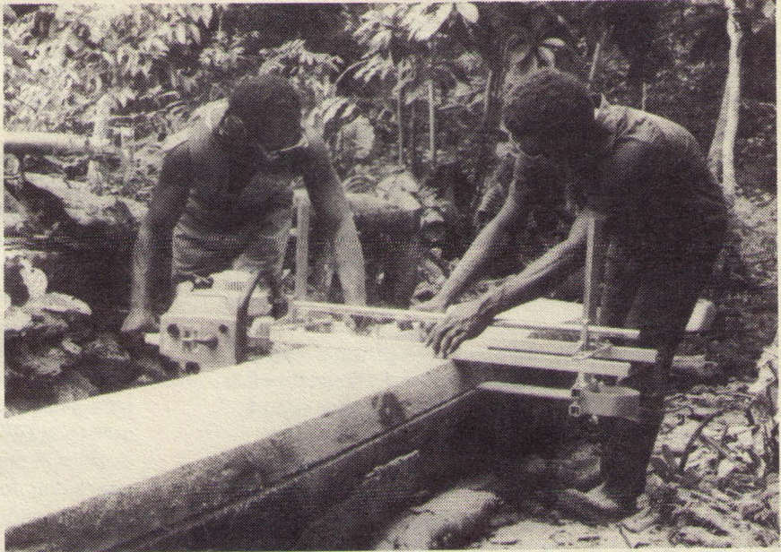
Joe Poniat and John Alto sawing a plank with the chainsaw and Alaska Mill Unit.
