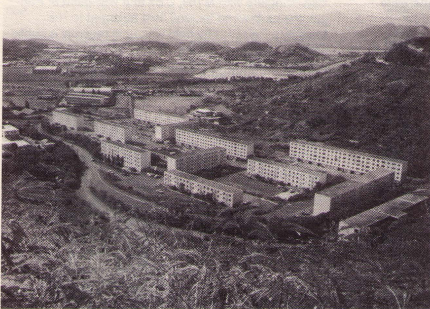
Low cost housing development on the outskirts of Noumea
