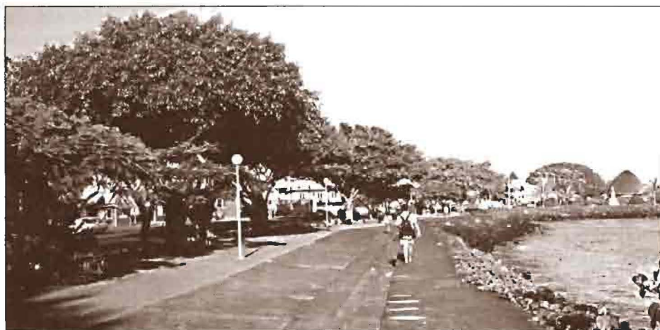
Walking along the volcanic rock and concrete constructed seawall in Apia, Samoa. To combat fears of erosion and as a first line of defense against storm waves and strong winds, several countries have built seawalls.
